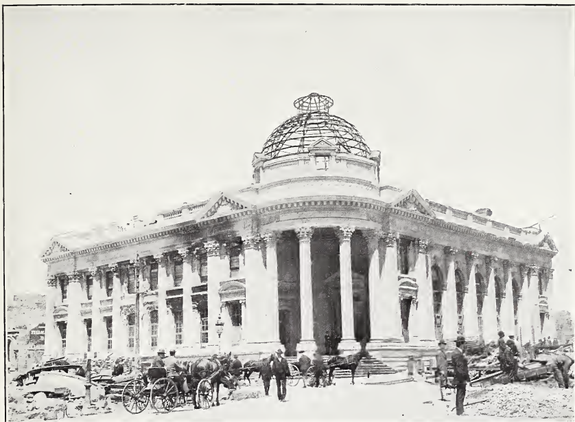
A. STONWORK SPALLED BY FIRE, HIBERNIA SAVINGS AND LOAN SOCIETY'S BUILDING, SAN FRANCISCO.
